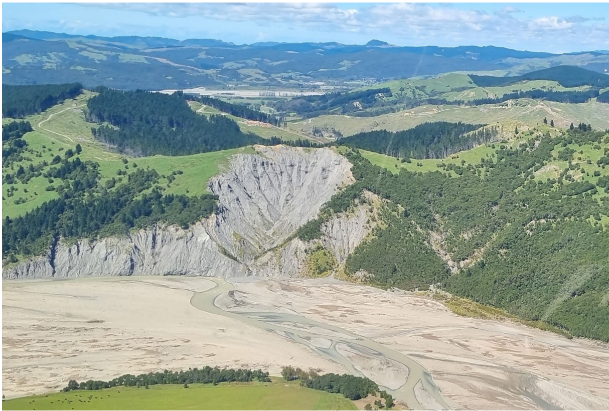
Figure 6: Untreated gully erosion, Tairāwhiti. “Gully Erosion is a cancer in the Waipū Catchment” (Mike Marden)
