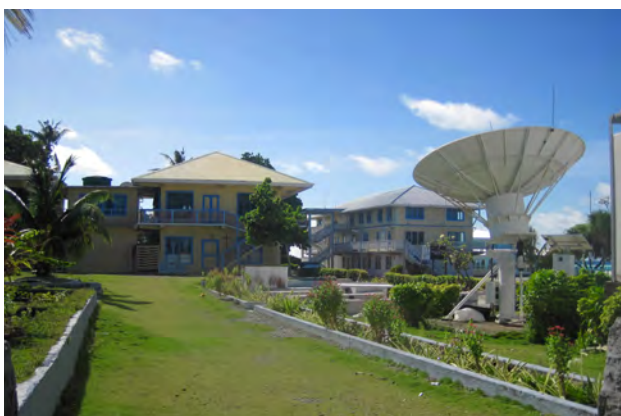
Telecommunications Infrastructure are critical lifelines for Tokelau Nukunonu, August 2016. Photo courtesy: C.L. Anderson.
