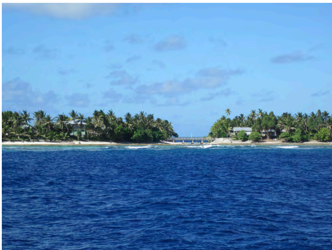
Coastal hazard mapping will consider risks to critical infrastructure, such as bridges. Nukunonu, August 2016. Photo courtesy: C.L. Anderson.
