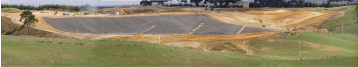
Cell 1 Hampton Downs under construction in 2005 (photo ref. EnviroWaste)
