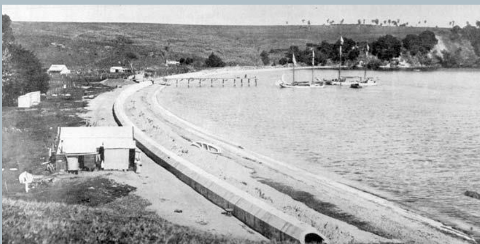
A sewer pipe under construction at Ōkahu Bay in 1910, in front of the ancestral village of Ngāti Whātua (buildings on left). Source: 7-A2929 Sir George Grey Special Collections, Auckland Libraries
