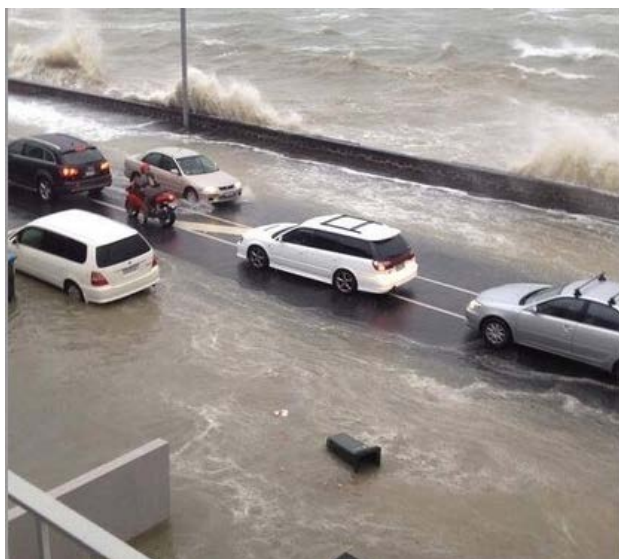
Figure 35: Inundation caused by wave overtopping of the seawall along Auckland's Tamaki Drive during ex-tropical cyclone Ita , 17 April 2014
