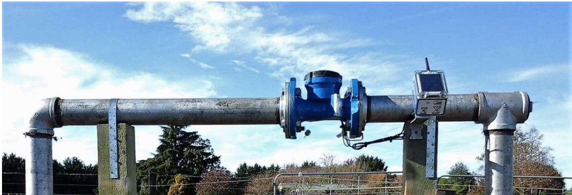
An ultrasonic water meter is connected to a solar powered telemetry unit.
