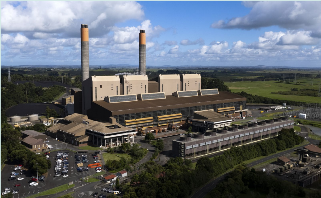
Image: Huntly Power Station
