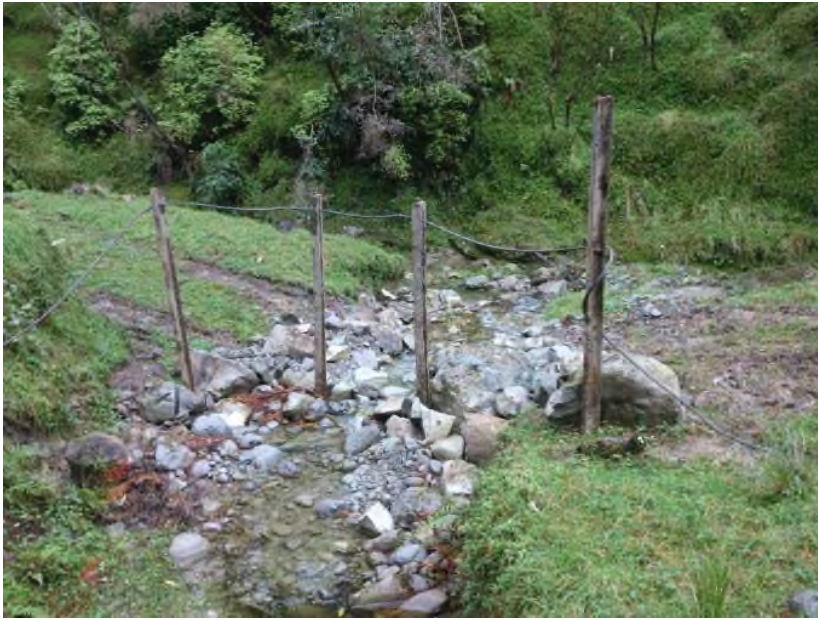
An example of a simple railway iron/cable debris trap anchored by deadmen.
