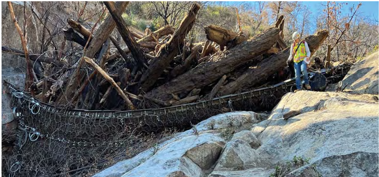
Figure 11 - VX barrier in New Mexico
