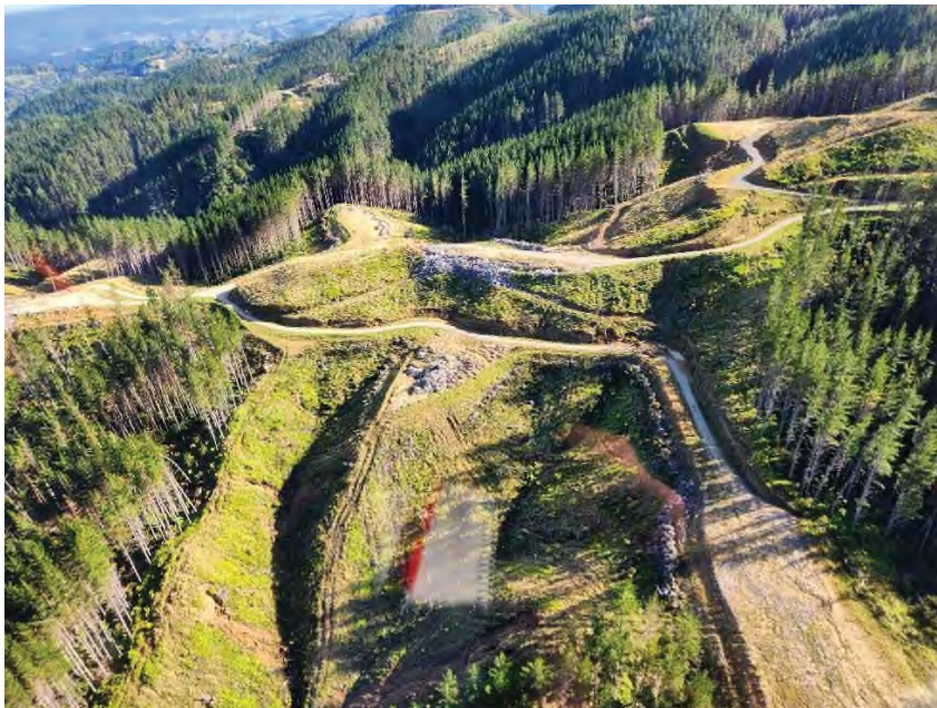
Post-Labour Weekend infrastructure construction. It was evident this held up well.
