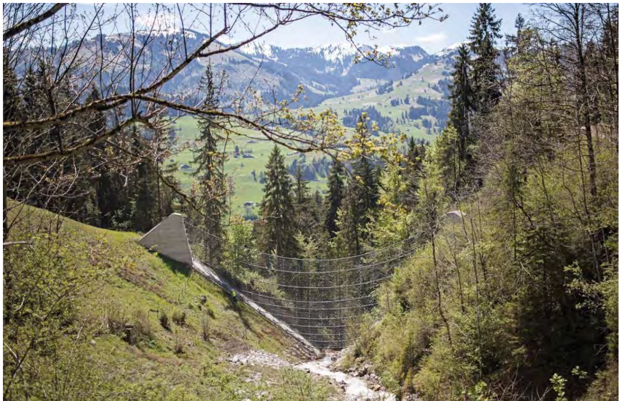
Figure 14 - Hüpach System 40m wide 10m high
