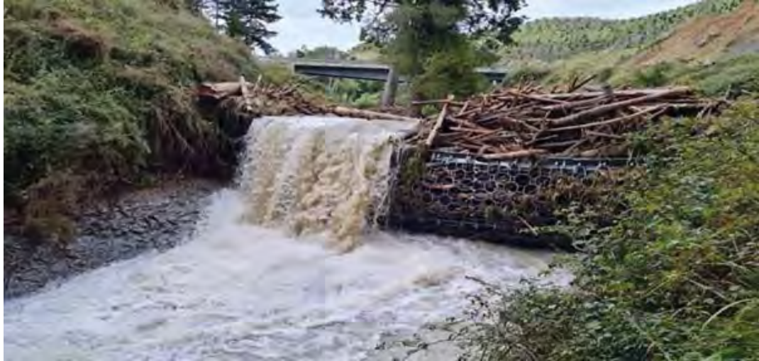
A well anchored debris net that has successfully trapped a large volume of large woody debris. The image is from a Hawkes Bay. The company has noted their effectiveness, with the trap catching debris in even smaller storm events.
