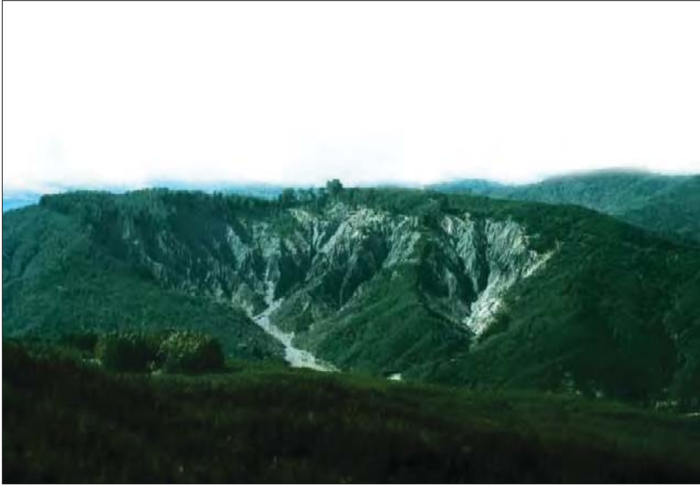
Photo2. The same area six years after planting. This illustrates clearly how quickly forest cover can be established and erosion contained.
